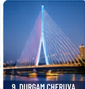
9. DURGAM CHERUVA CABLE BRIDGE
