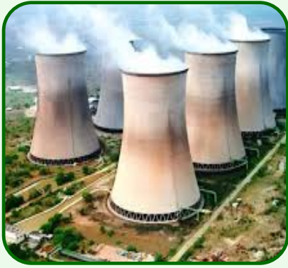
Thermal Power Station
